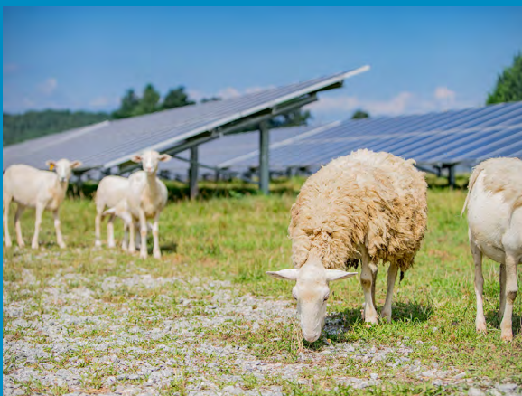
Right: MT Olive Solar 1 site (6.5 MW; Wayne County, NC
