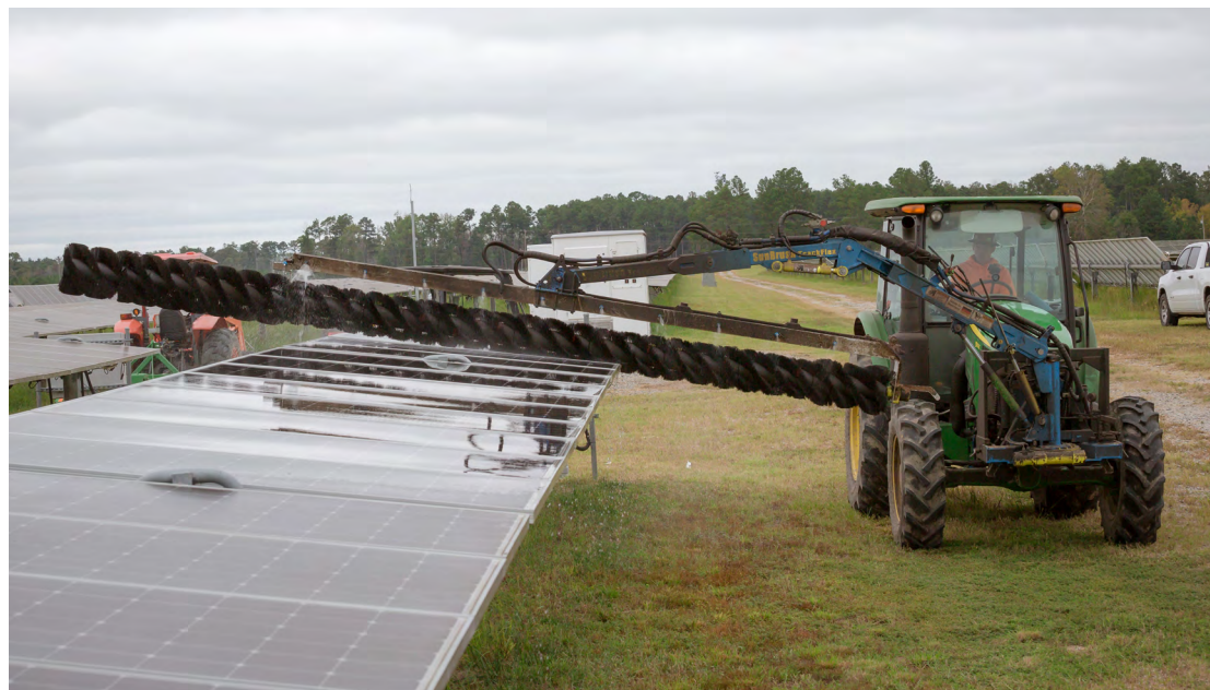
Module washing at our Shoe Creek Solar facility in North Carolina
